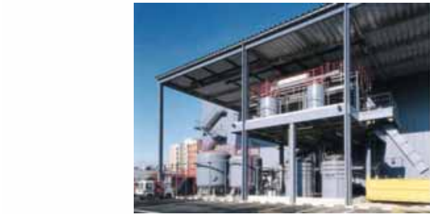
Waste water treatment facility. Fine dust or dirt in water used for washing products are removed at the water treatment facility and the restored discharged water is so clean that fish thrive in it.
