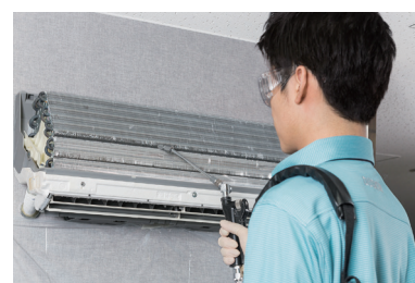
Cleaning air conditioner for residential/ commercial use
